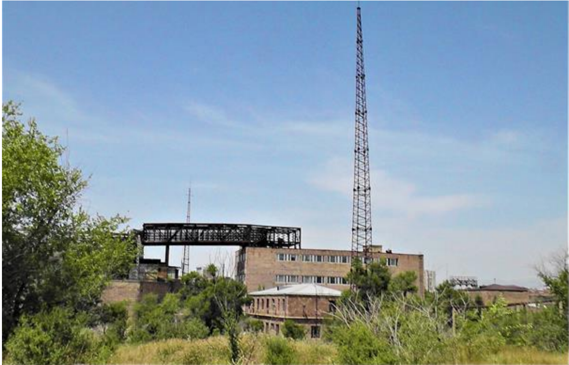
In the foreground is the building of LUE-75
